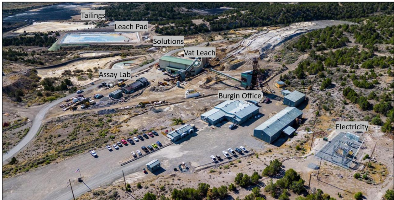
Figure provided by Osisko Development.
