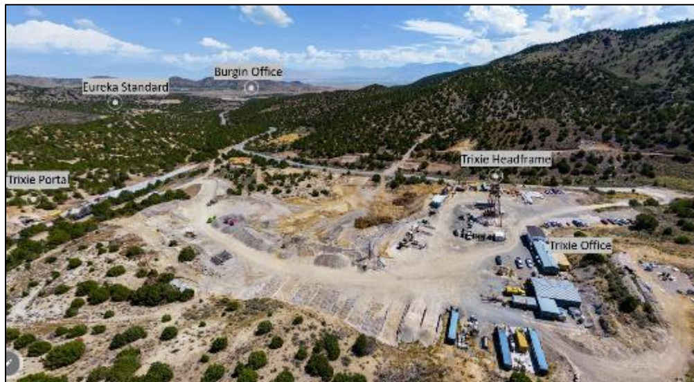
Figure 5.1 Overview of the Trixie Test Mine looking towards the Northeast
