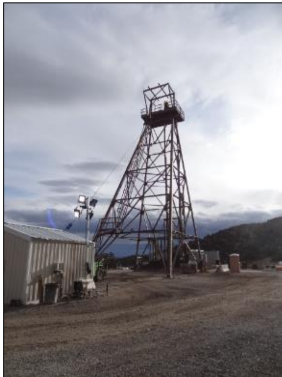
Micon 2022 site visit photograph.
