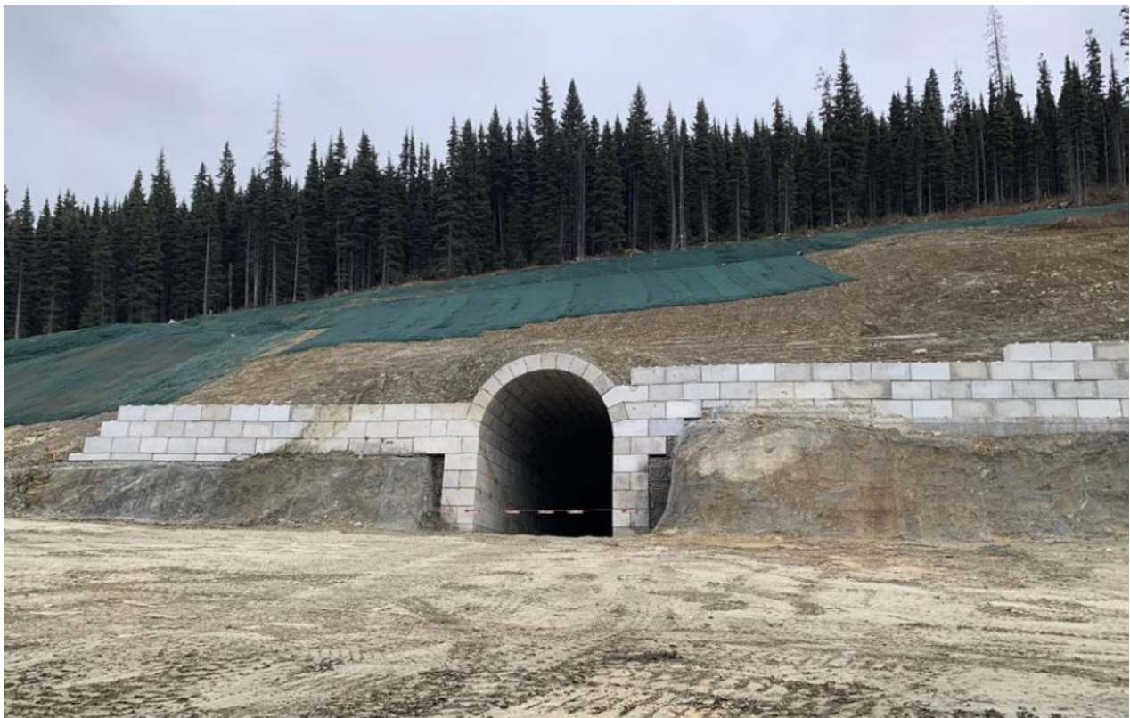
Figure 16-7: Cow Portal shortly after construction
