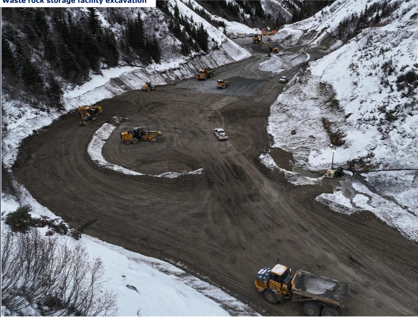
Waste rock storage facility excavation
