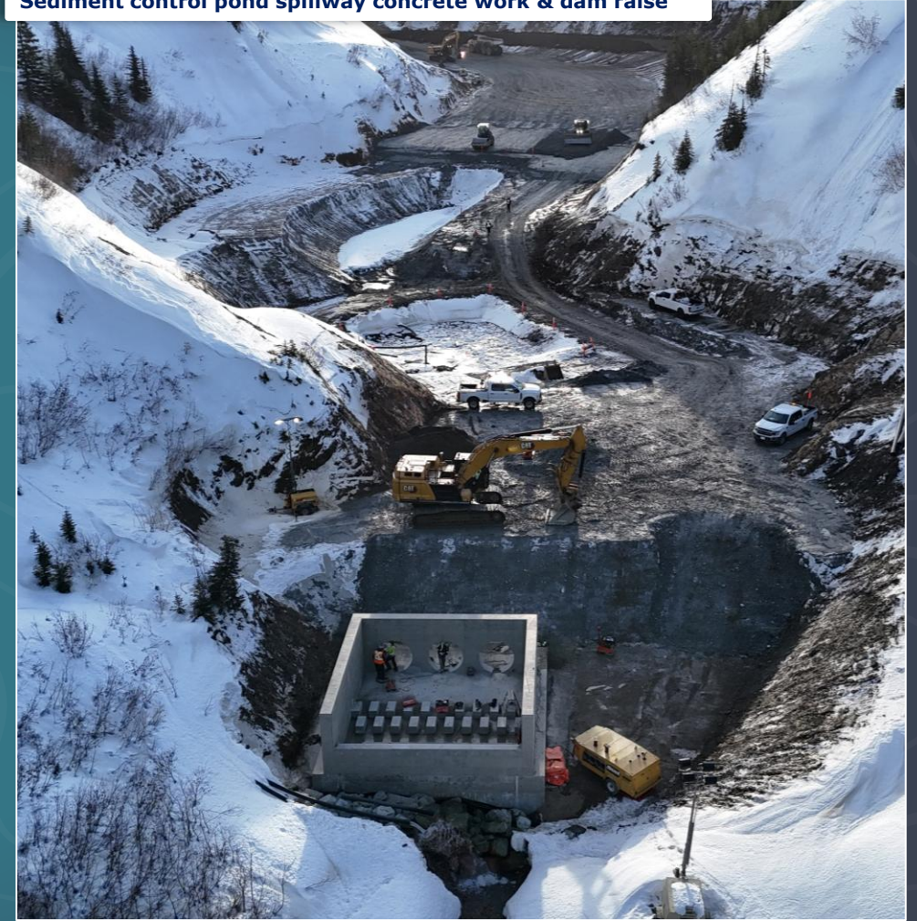
Sediment control pond spillway concrete work & dam raise
