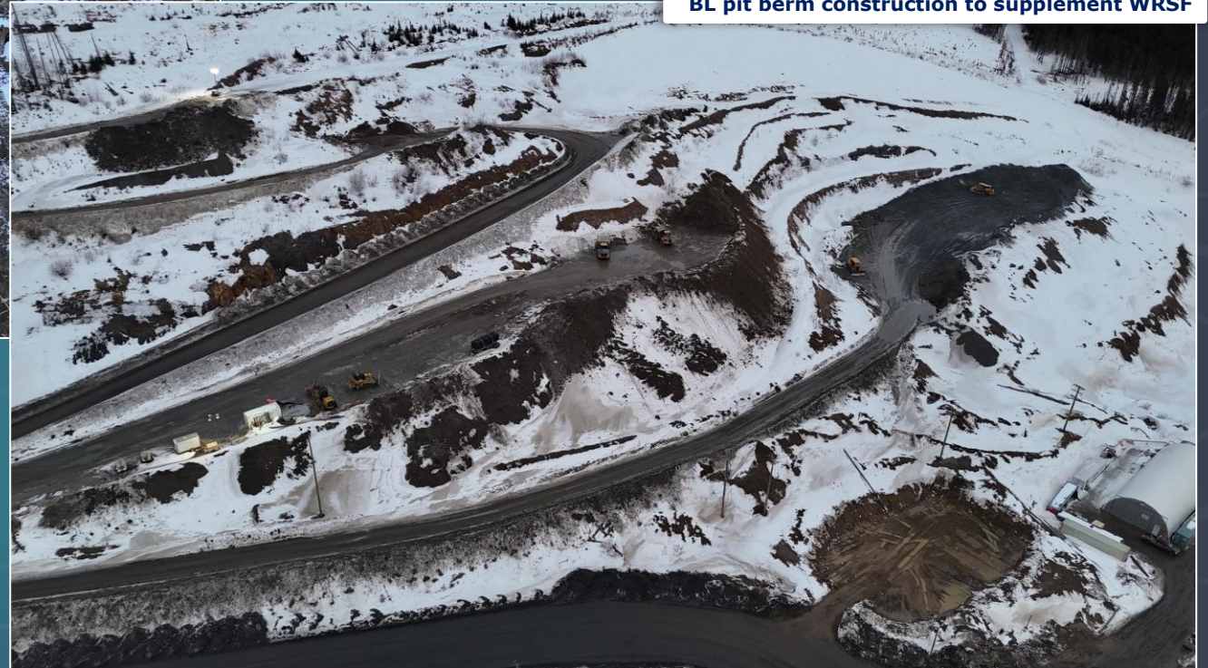
BL pit berm construction to supplement WRSF
