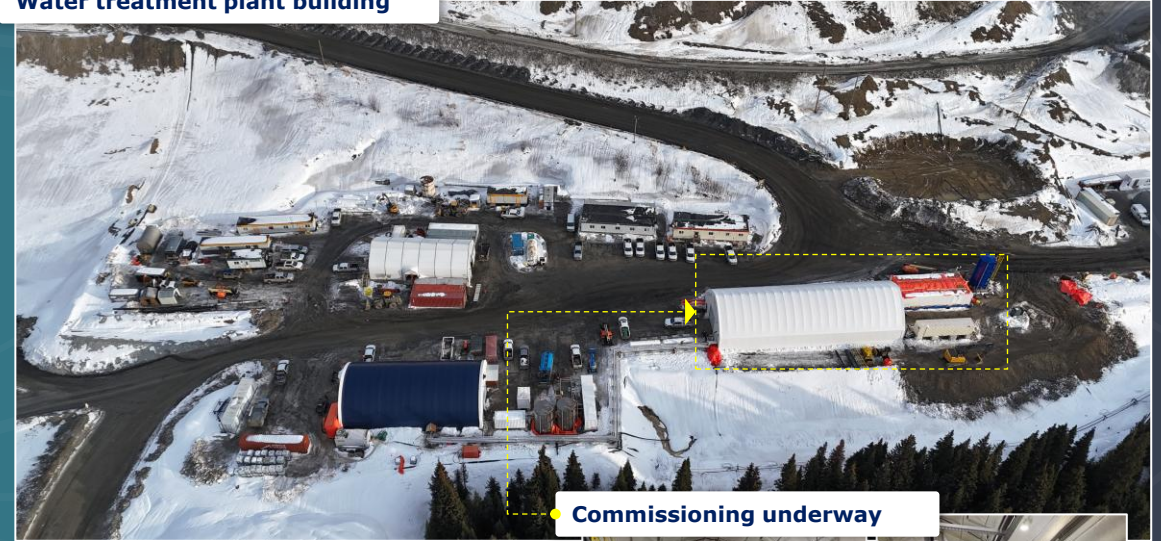
Water treatment plant building
