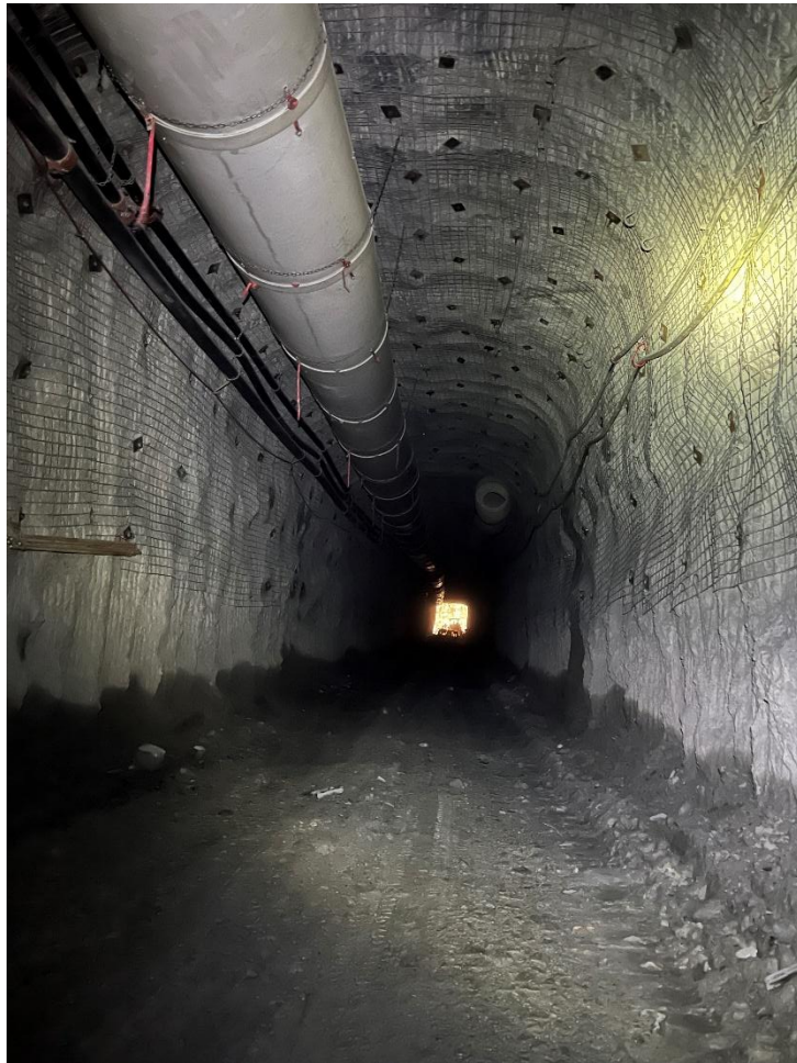
Figure 6: Main decline ramp from Cow portal (5.4 meters wide x 5.8 meters high).
