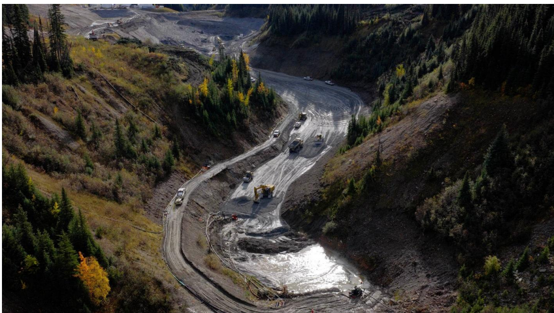
Figure 3: Sediment control pond (SCP) stripping in progress.
