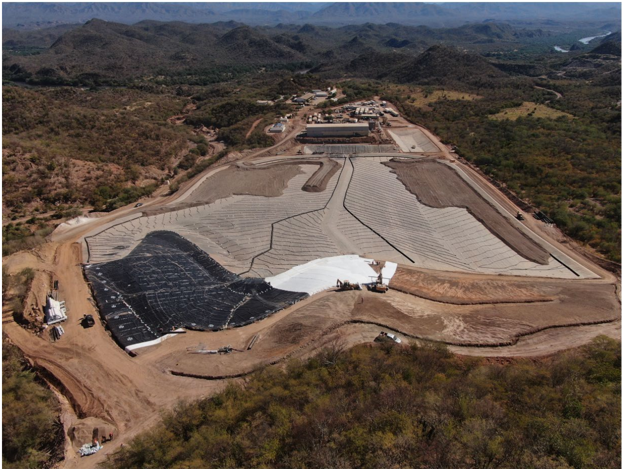
Figure 1: San Antonio Oxide Stockpile – Leach Pad Construction
