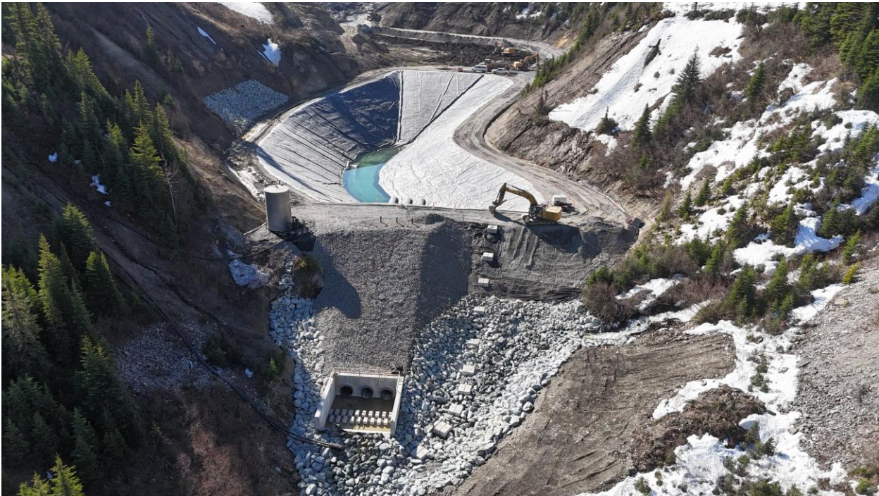
Figure 2: Sediment control pond (SCP) installed liner and placement of aggregates.
