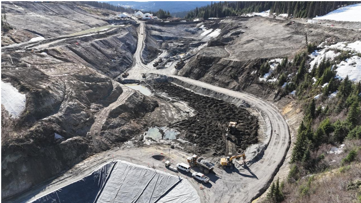
Figure 1: Waste rock storage facility (WRSF) aerial overview of ongoing works.
